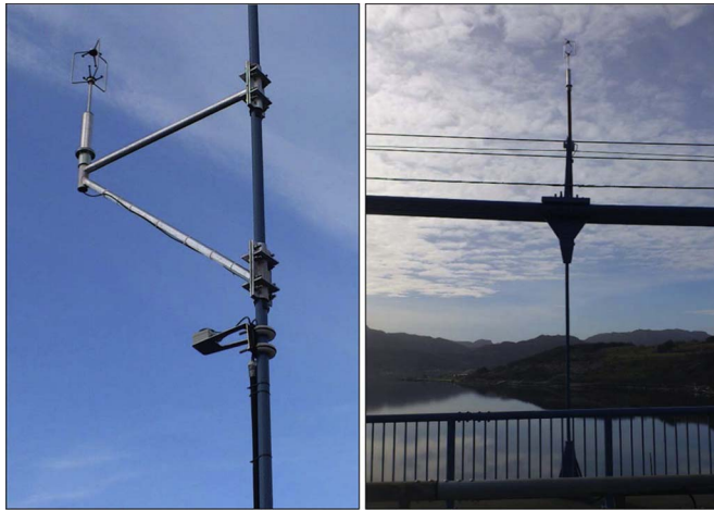
Fig. 4. Sonic anemometer fixed at a hanger (left) and at the top of a pole (right) at Lysefjord Bridge.
